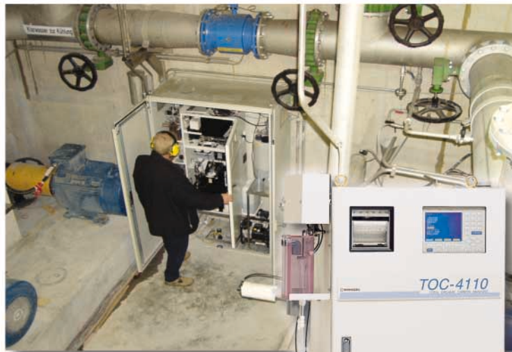
Figure 7: Location of the TOC-4100 online analyzer (on the right: The next generation: TOC-4110)
