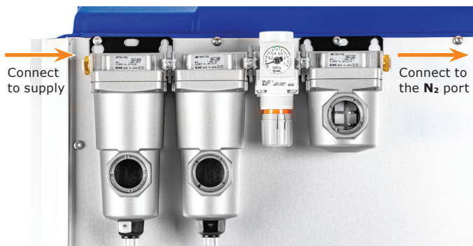
Figure 69. The setup of the filter unit for the N 2 port.
